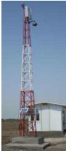
Tower with PTZ camera, Monitoring unit and Data Logger for Wireless Sensors, Wi-Fi Internet, etc.
